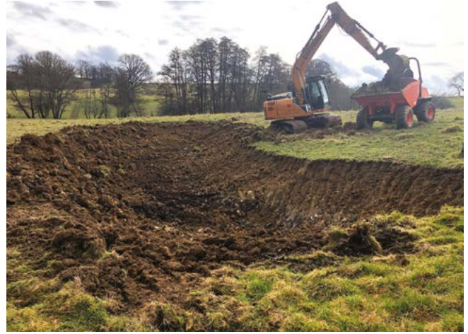
Fig. 32. ‘Ghost’ pond restoration requires careful excavations.
