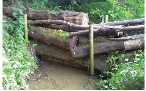
**Fig 9.** Bottom log partially collapsed and logs above now fallen or unstable
