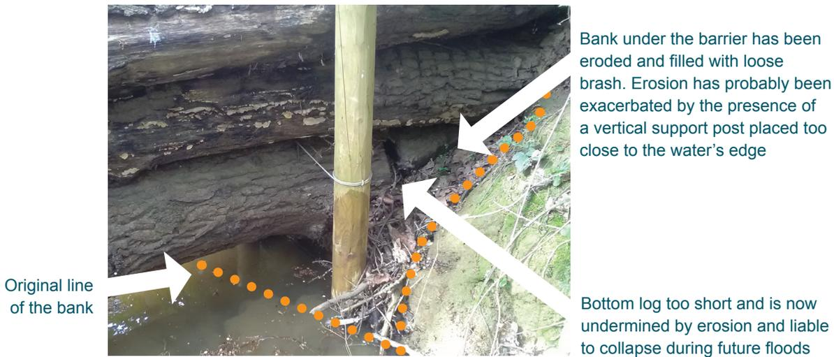
**Fig 6. Bank erosion / embayment**
