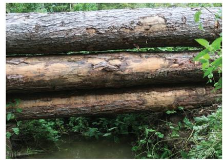
**Fig 2.** Larger gaps below and between the leaky barrier logs are designed to ensure they rapidly drain away flow from preceding rain events creating greater storage capacity for large floods
