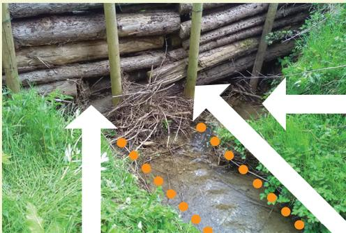
Bottom log has fallen into the channel upstream of the barrier because the bank into which it was embedded has been eroded. The log now blocks normal flows
