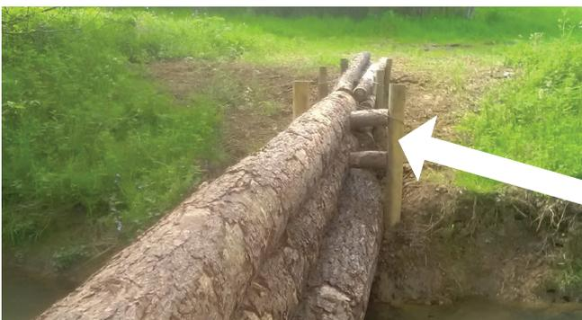
Horizontal batons are needed here to brace the upper logs against the vertical support post because the lowest log is wider than those above. This is not an optimal solution and it is not clear how well the batons will persist in the longer term.
