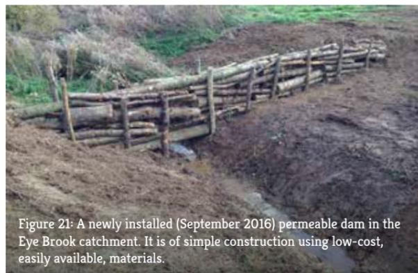
Figure 21: A newly installed (September 2016) permeable dam in the Eye Brook catchment. It is of simple construction using low-cost, easily available, materials.
