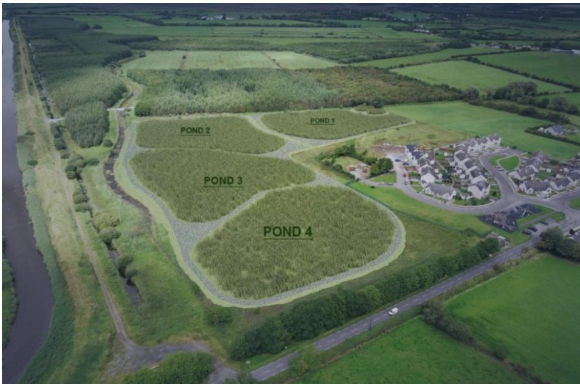
Figure 13. Before and after views of a new constructed wastewater treatment system in Lixnaw, Co. Kerry which cost £1.72 million.
