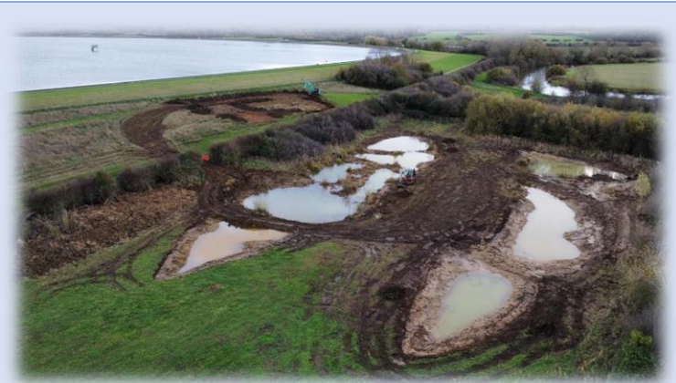
15 Contractors working on Buckthorn Meadow
