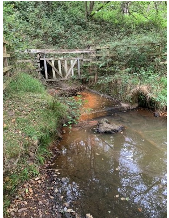
The current structure at Ocknell Arch
