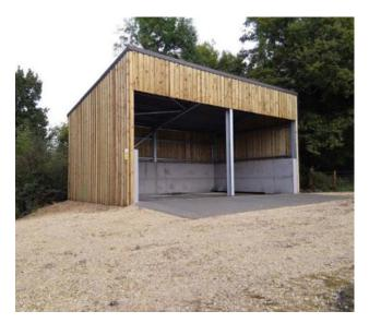
This manure store was constructed to prevent the leaching of nitrates and phosphates into the nearby stream and a rainwater collect tank was installed on the far side.
