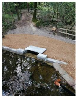
The eel pass at Middle pond where adjustments and maintenance work has been carried out to keep the pond accessible to eels.
