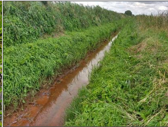
Ochre stained section of dyke with no aquatic plants
