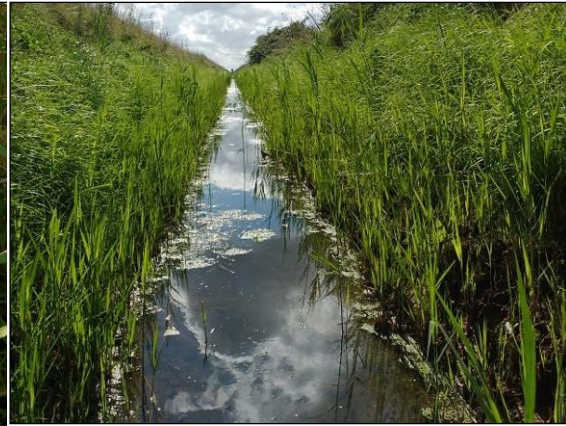
Open channel and regrowth on bank face in August
