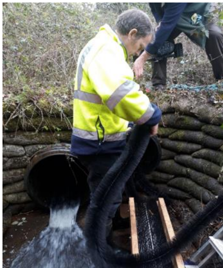
Fitting the gutter brush and eel ramp at Boarman Pond.
