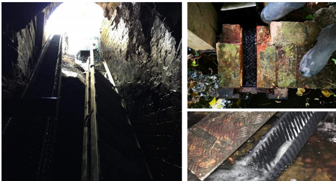
Newly installed eel pass disappearing into the depths of the culvert which carries the Hartford Stream underground from the Stew Pond in the grounds of the Beaulieu Abbey to the top of the Beaulieu Estuary. The bottom right picture also shows the toe of the otter ramp which was reinstalled above the eel pass.
