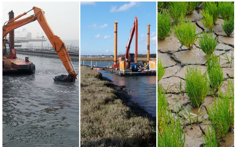
Pilot project: Beneficial use of Dredging's, Lymington. Photo courtesy of ABPmer
