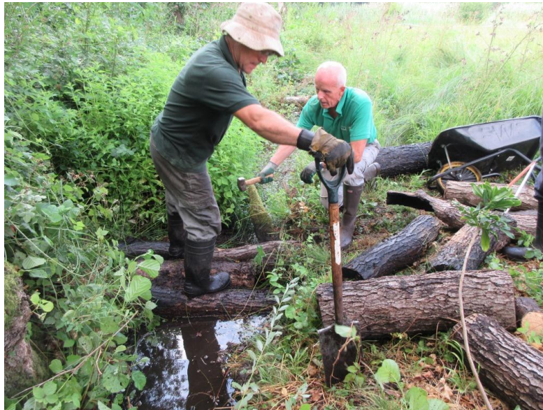
Reversing historic drainage: volunteers installing a partially leaky log dam in the outflow drain from the Ruskin Reserve in July 2018. Photo J. A. Webb.
