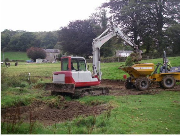
Figure 3. Left: Tracked digger constructing ponds and dumper being used to take spoil away. Right: Spoil was spread in a depression in the adjacent field used for grazing small numbers of livestock.
