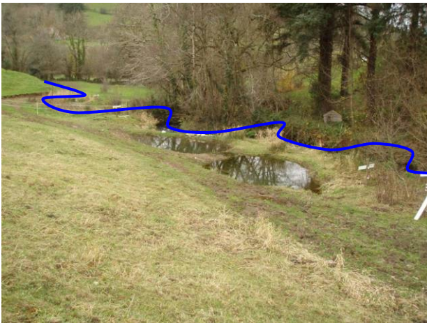
Figure 4. Left: Constructed ponds in line with the Nant Eion (blue line). Right: The pictures show ponds holding water a few months after creation. Small size and shallow depth was important for attracting breeding amphibians.
