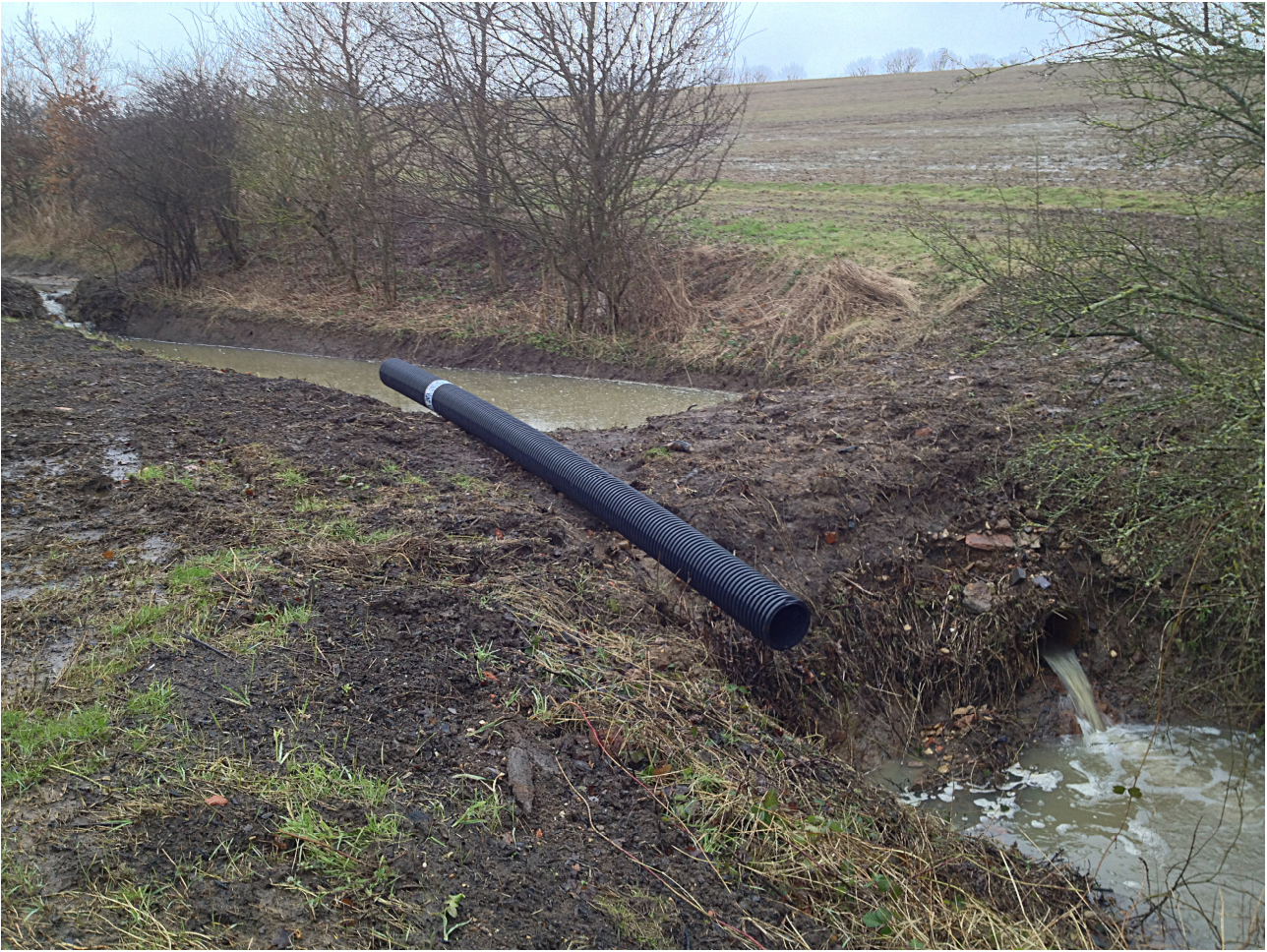
Figure 56. Large earth banded ditch interceptor under construction.
