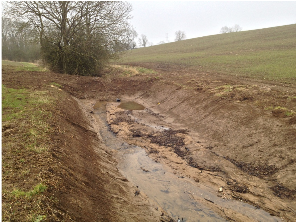
Figure 51. Large earth bunded ditch. The picture shows the bund before being 'switched on', with bottom pipe still open. This pipe is now closed and the bund retains water and sediment during high flows. Note that the photograph was taken before the top pipe was installed.
