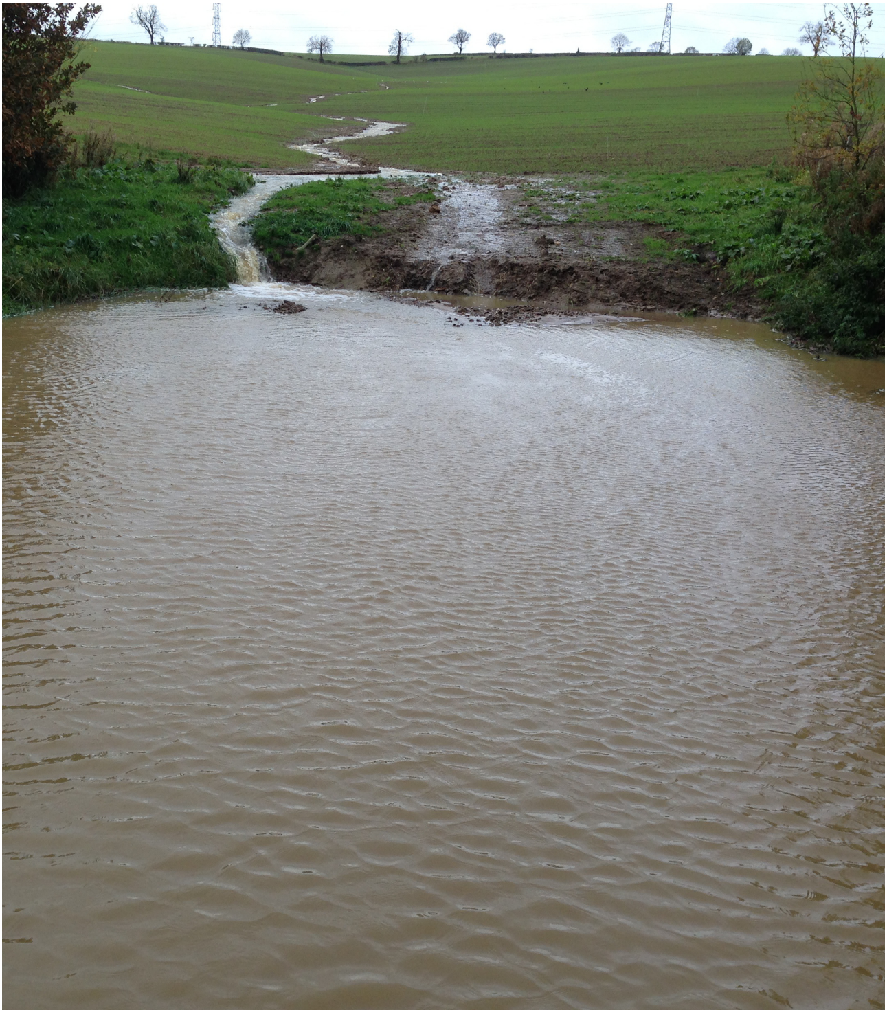
Figure 53. Field drain interception ponds. The picture shows a pond intercepting a field drain that previously discharged directly into the Eye Brook (behind photographer). This drain collects water from a field which represents about 5% of the arable area in Eye Brook project area. Note that there was overland flow and gullying along the line of field drain because the drain was too small to take the flows occurring at the time of the photograph (January 2013). This field drain was replaced with a larger diameter pipe in autumn 2014.
